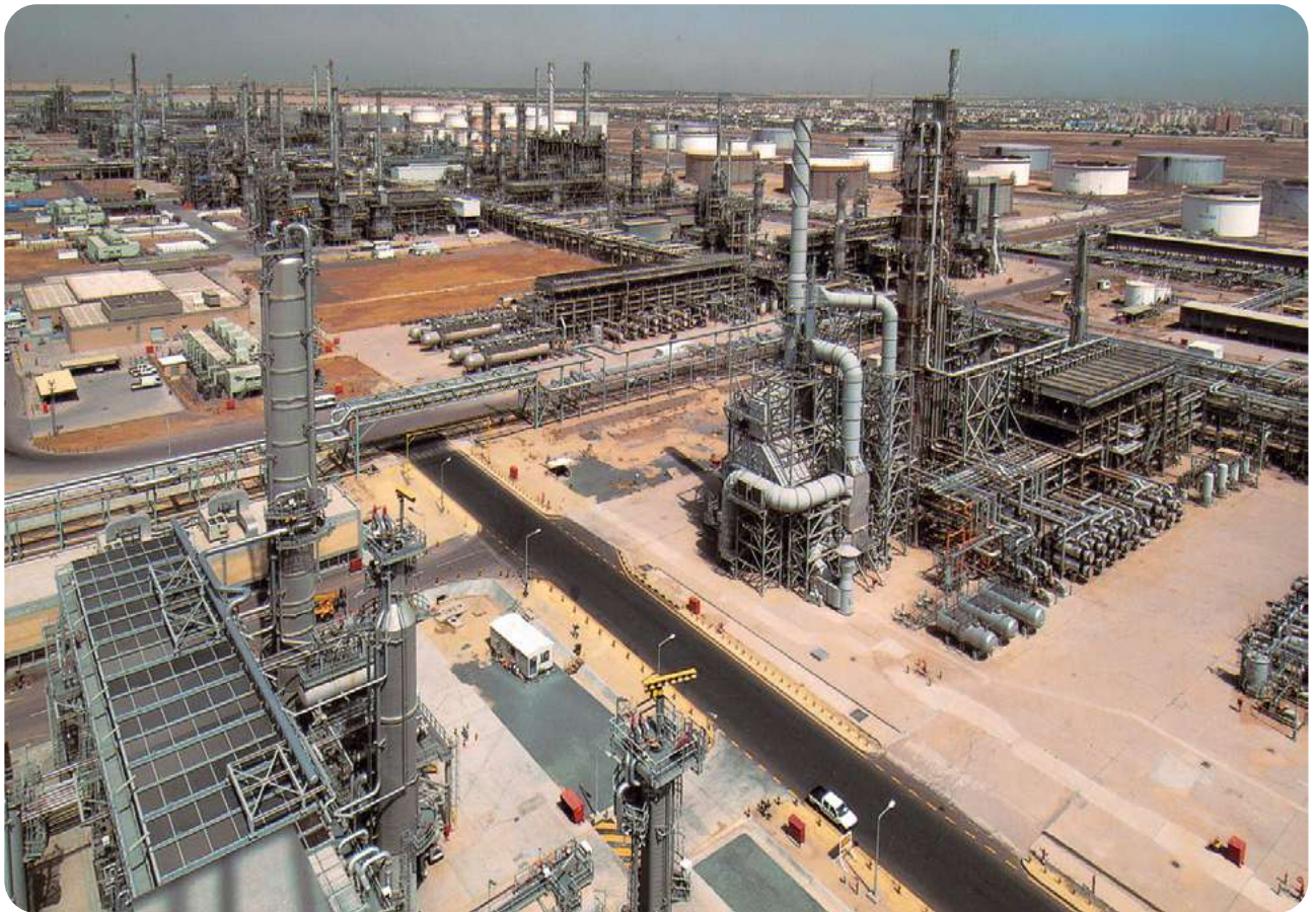
Mina Al Ahmadi Refinery Following the Rehabilitation
