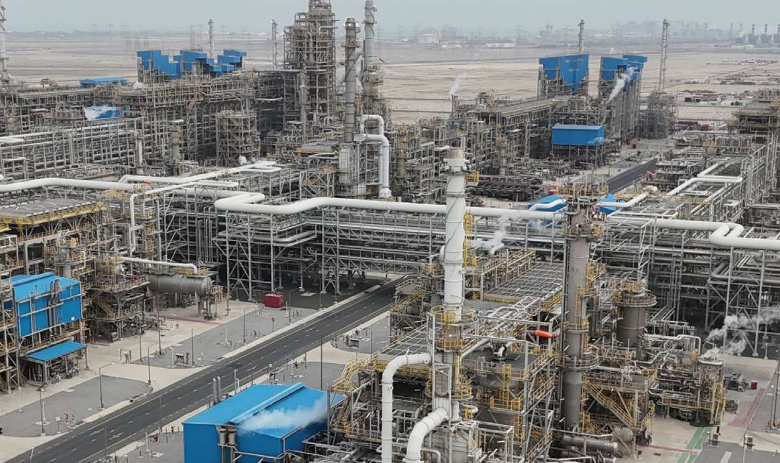
A View of Al-Zour Refinery Units
