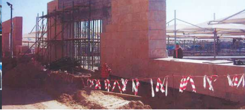
Construction Phases of the New Head Office
