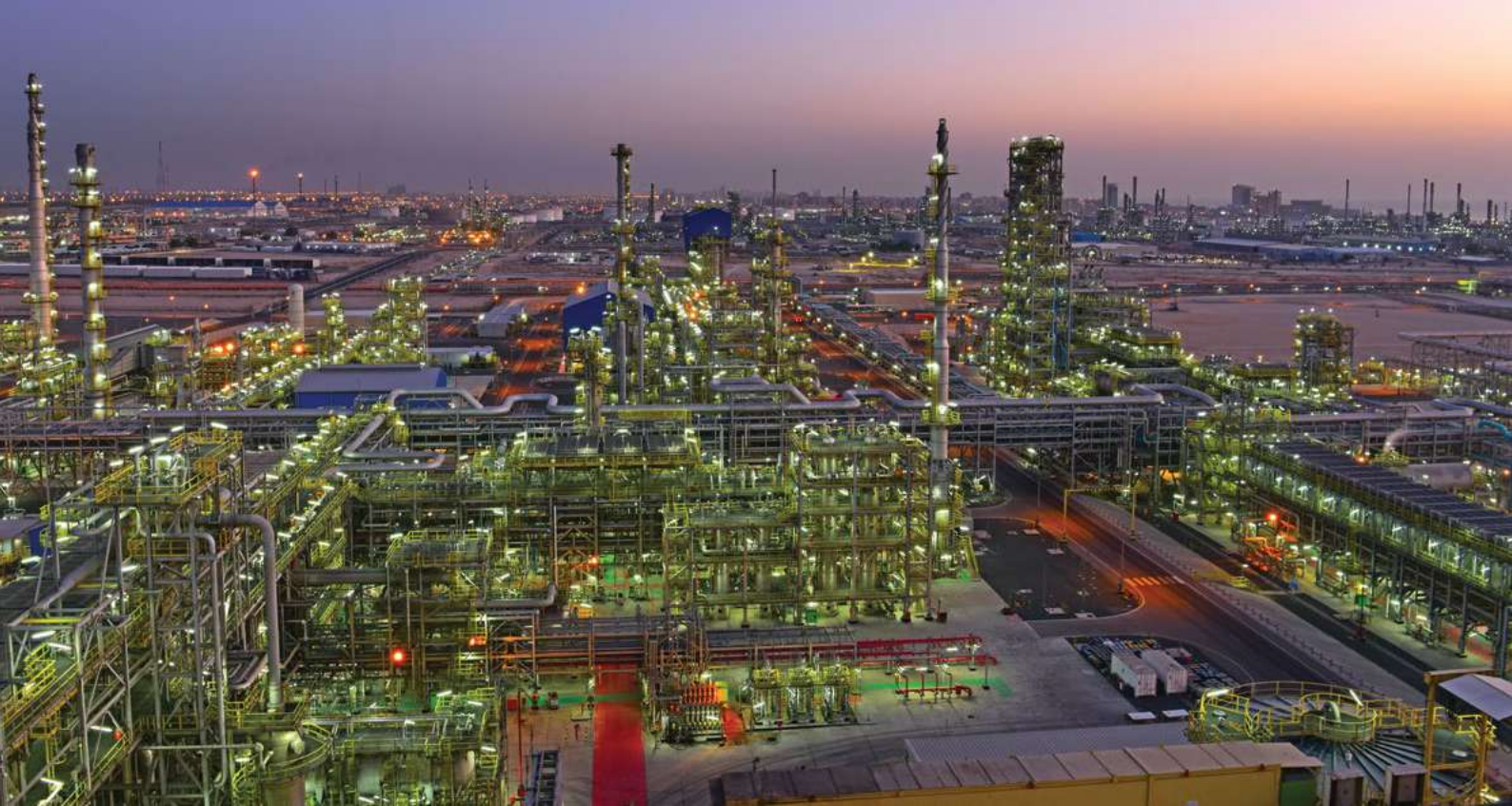
A view of the Clean Fuels Project after Completion
