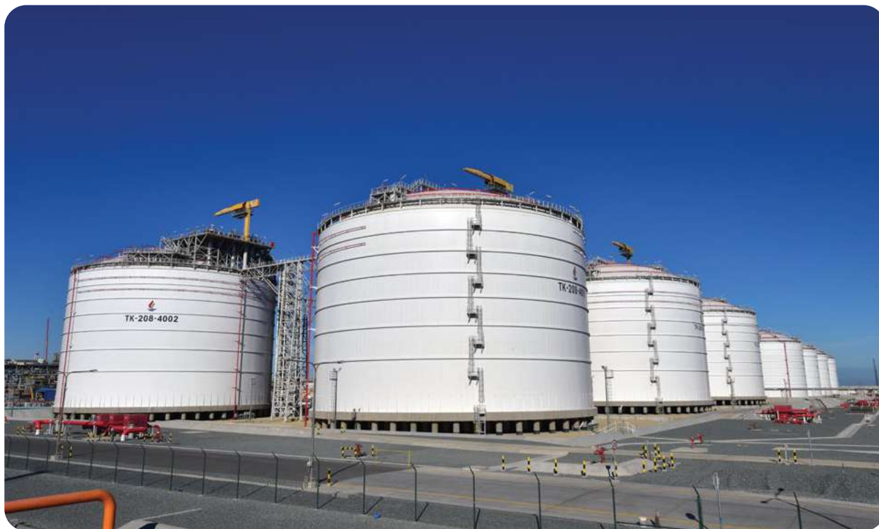
Northern Liquefied Gas Tanks
