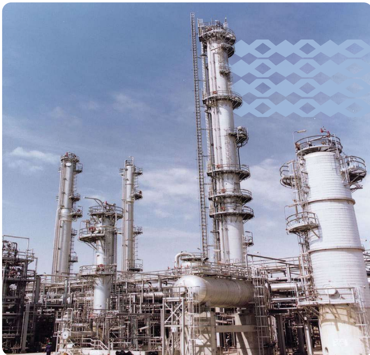
Jet Fuel Production Unit at Mina Al-Ahmadi Refinery
