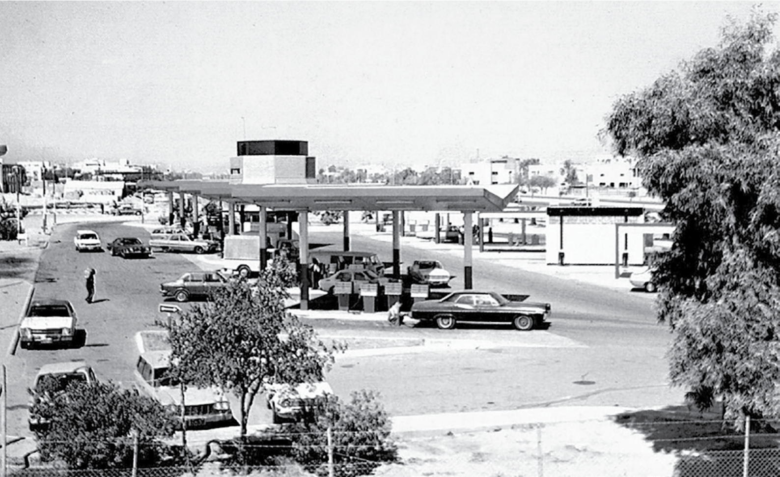
Old Fuel Station in Mansouriya Area
